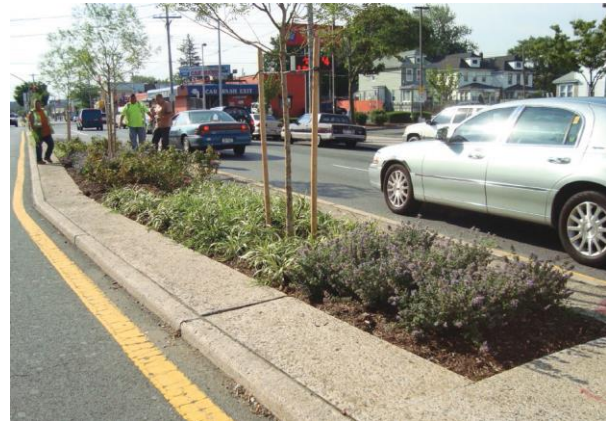
Curb-height median with plantings set back from the curb to allow for easier maintenance: Merrick Boulevard, Queens, New York. Source: NY DOT Street Design Manual
