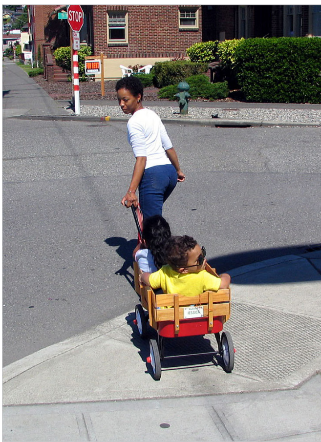
Figure 3.4: Example of a curb ramp www.pedbikeimages.org/burden
