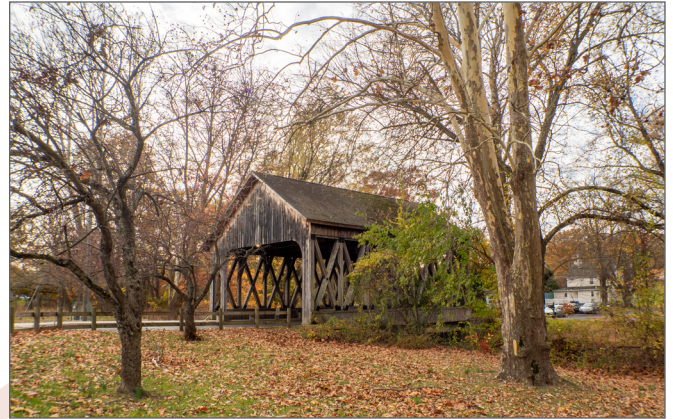
Figure 1.6: Twin Brooks Park covered bridge, Trumbull Colliers
