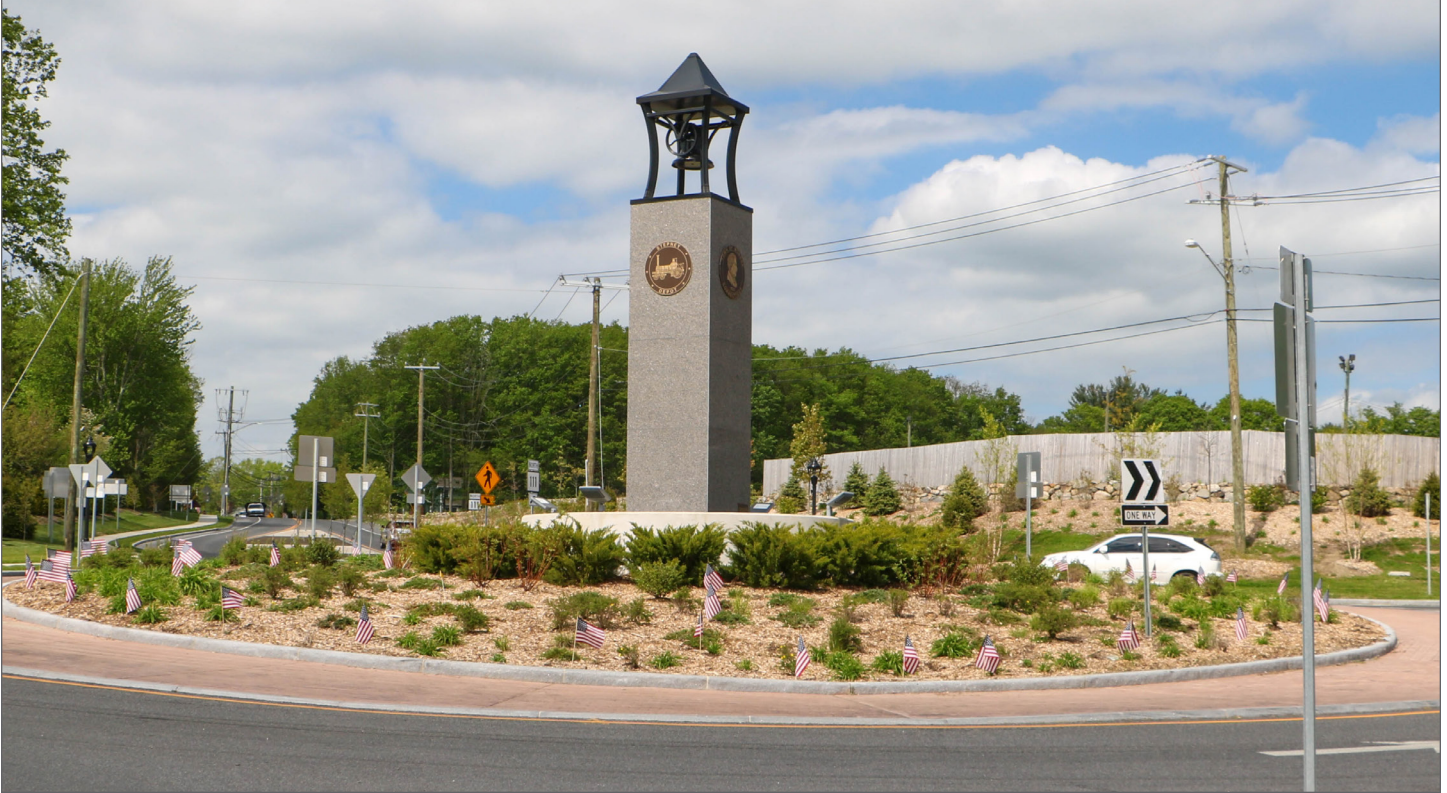
Figure 3.9: Route 111/110 Roundabout, Monroe
