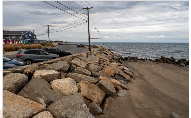
Figure 2.11: Long Beach Seawall, Stratford Colliers
